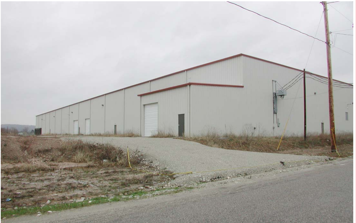
SOUTHWEST VIEW OF BUILDING
