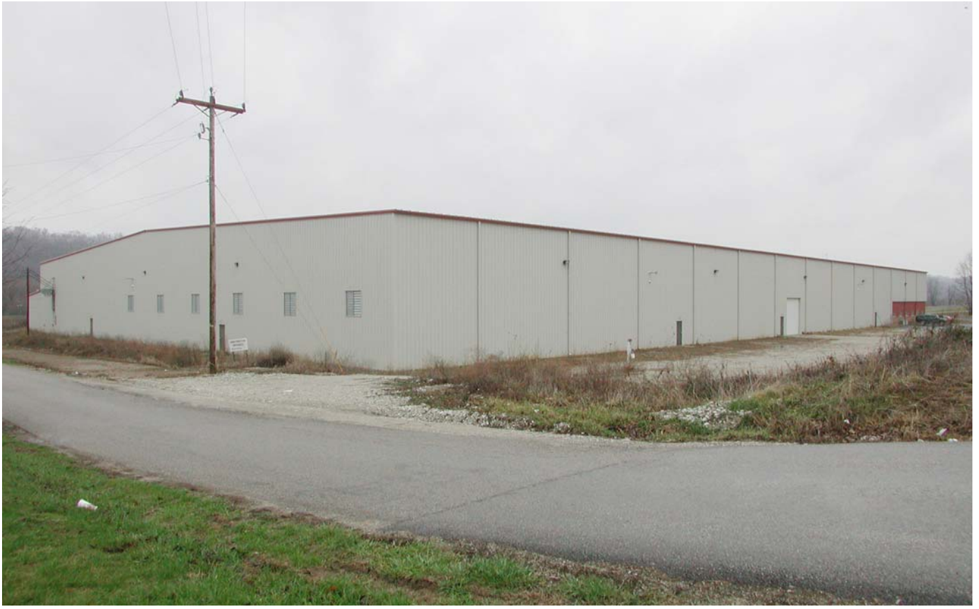
SOUTHEAST VIEW OF BUILDING
